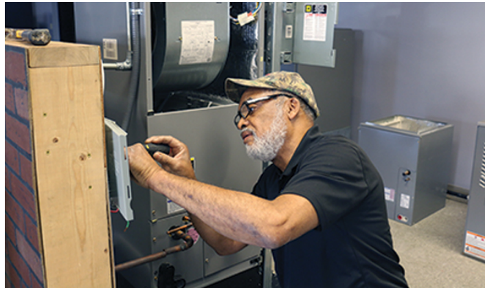
James Perkins installs a furnace in Remington College's new HVAC lab.
